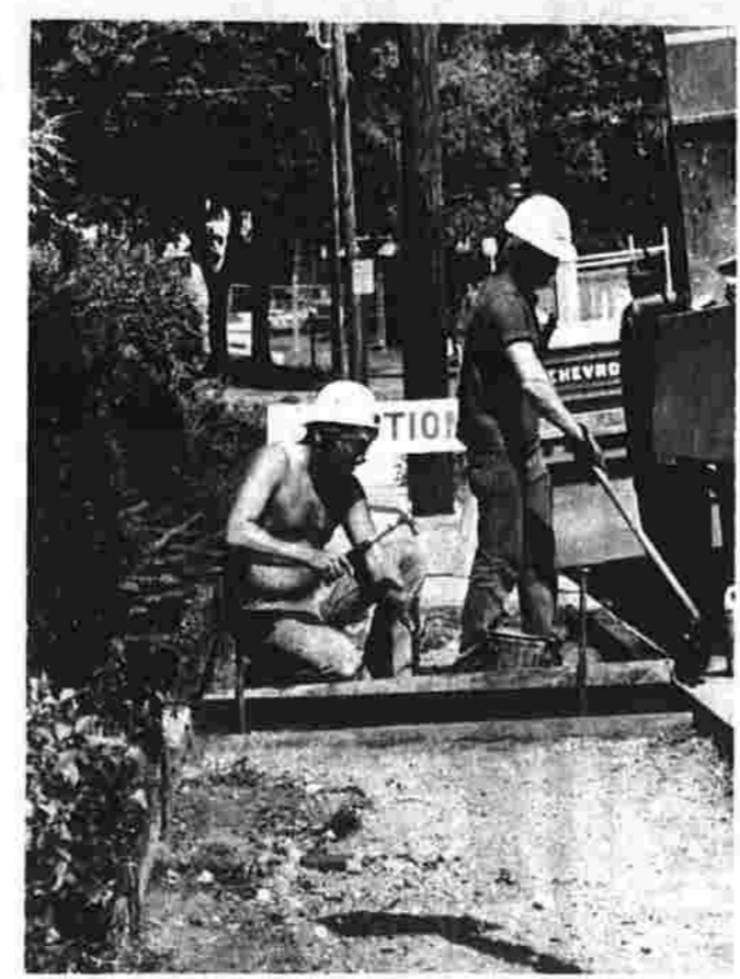
Sidewalk repair crew at work
